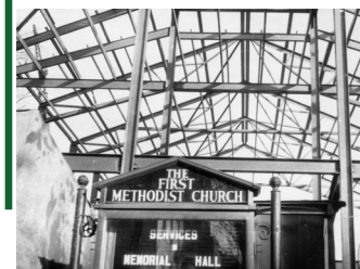
Athens FUMC being rebuilt
